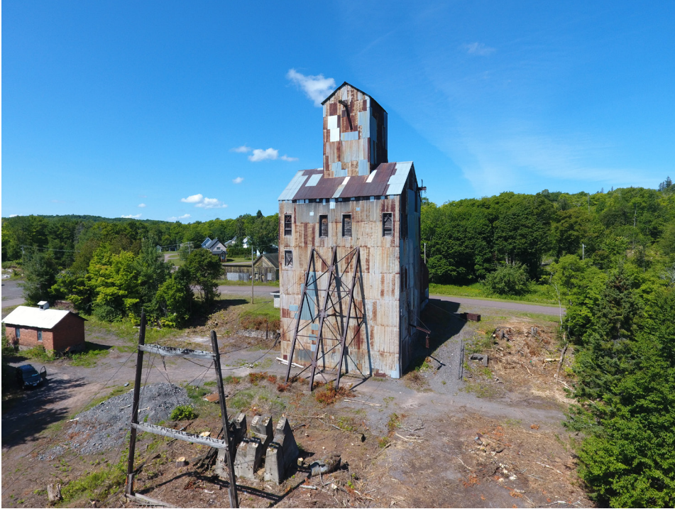
The shafthouse after the vegetation removal.
